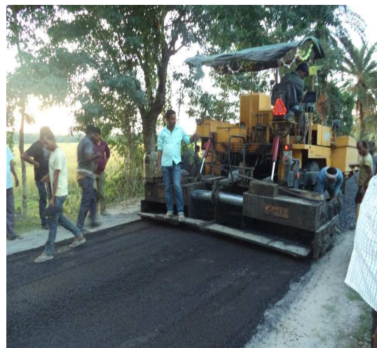
Figure 7: Laying & spreading of cold mix
