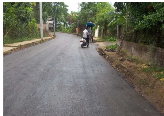
Figure 9: Completed cold mix road
