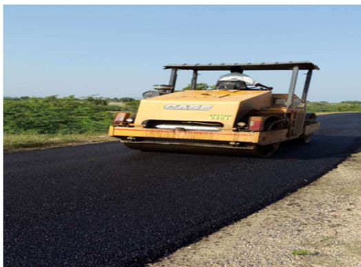
Figure 8: Compaction of cold mix surface
