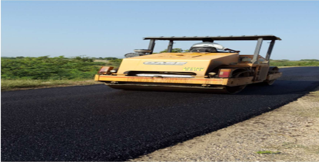
Figure 8: Compaction of Cold Mix SDBC surface by Roller
