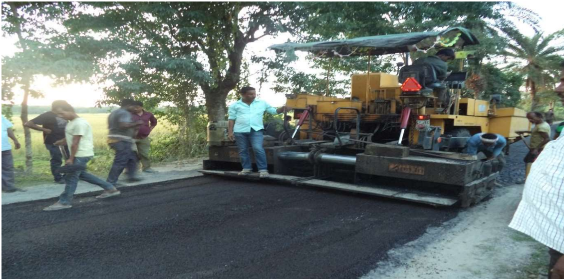
Figure 7: Laying of Cold Mix SDBC by Paver
