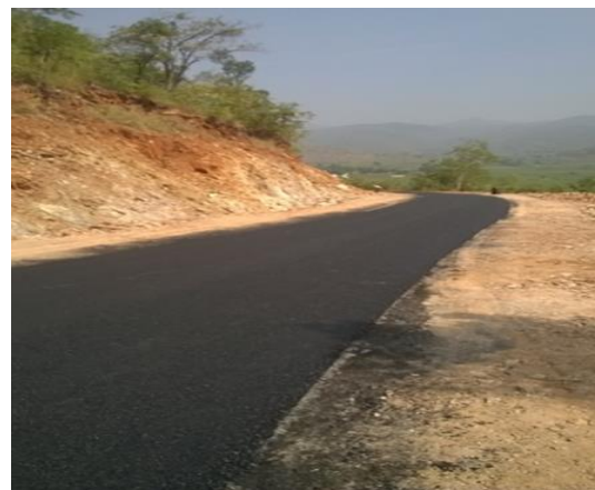
Image-10, completed CGPC road
