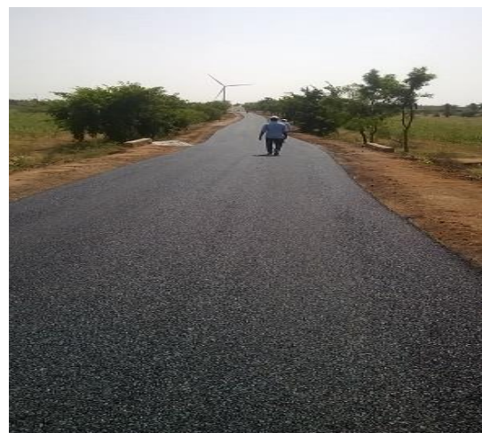
Image-8, completed CGPC road
