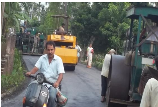
Image-14, laying & compaction cold mix SDBC
