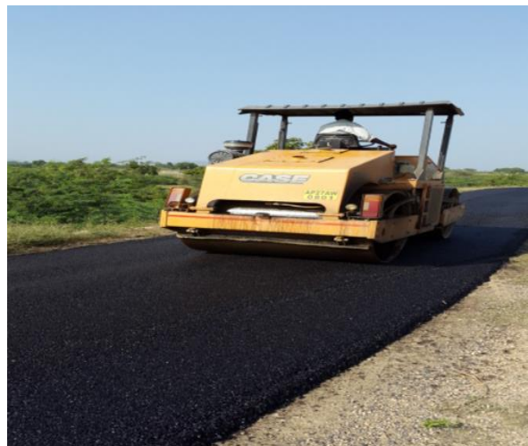
Image – 13, compaction of cold mix MSS
