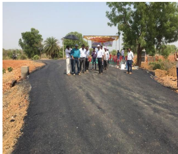
Image-17, completed seal coat surface
