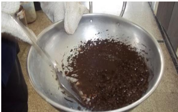
Image-3, preparing cold mix SDBC Image-4, prepared mix is kept on to a tray
