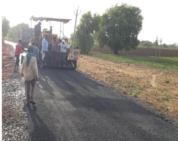
Image-16, laying of cold mix seal coat
