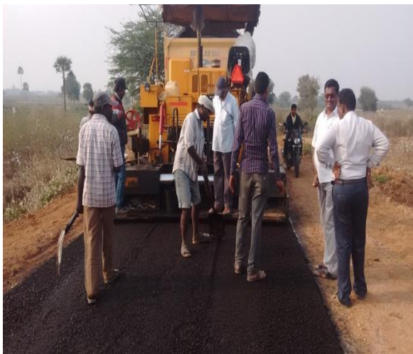
Image – 12, laying of cold mix MSS
