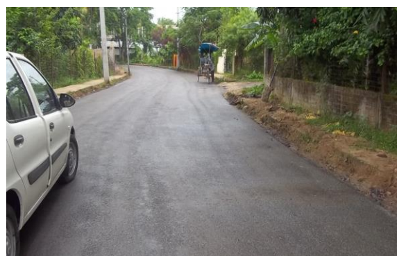
Image-15, completed cold mix SDBC road
