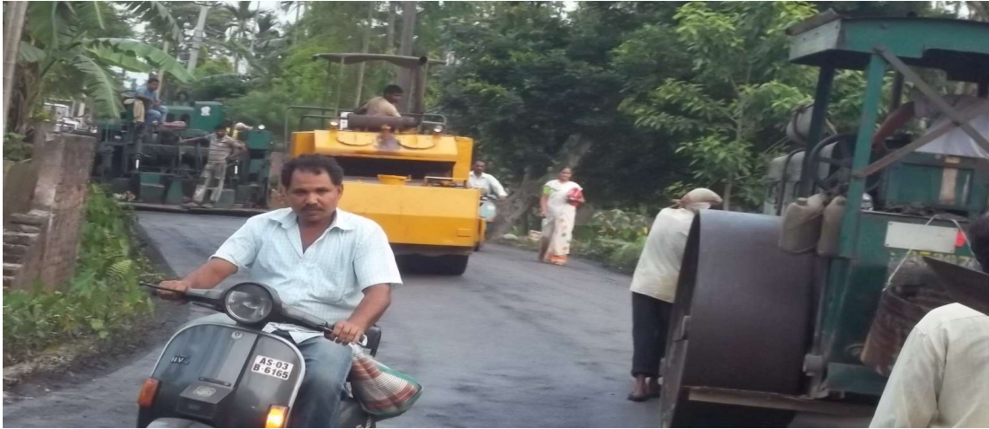
Fig 12 Cold Mix SDBC laying by paver and compaction by roller
