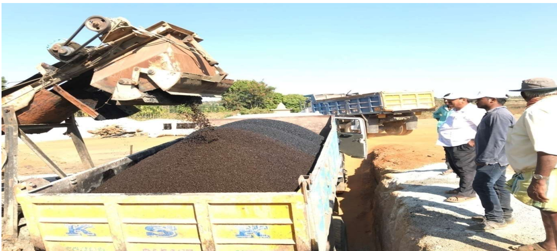
Fig 11: Cold Mix SDBC Production through converted Hot Mix Plant
