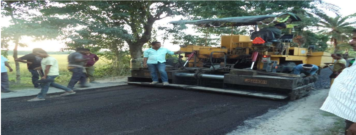
Fig. 9: Laying and spreading of cold mix CGPC by paver
