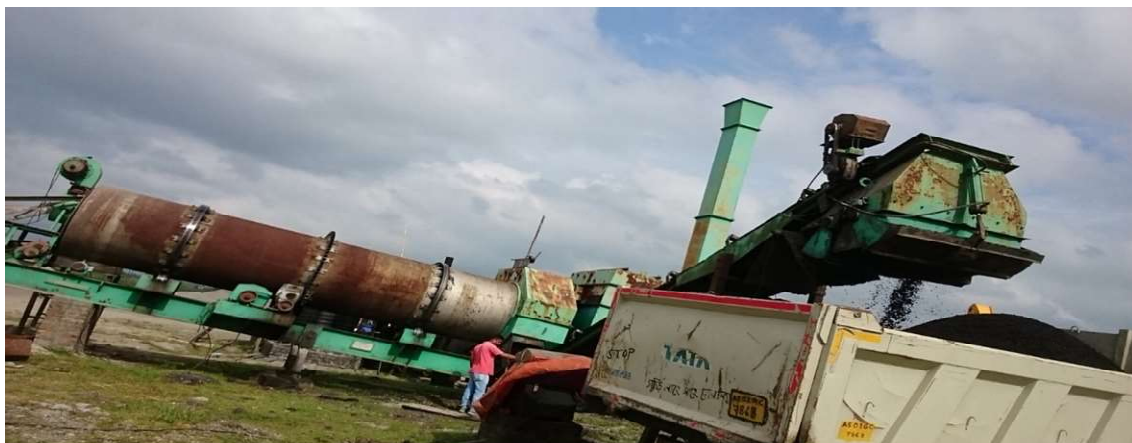
Fig 8: Cold mix CGPC production through converted Hot Mix Plant
