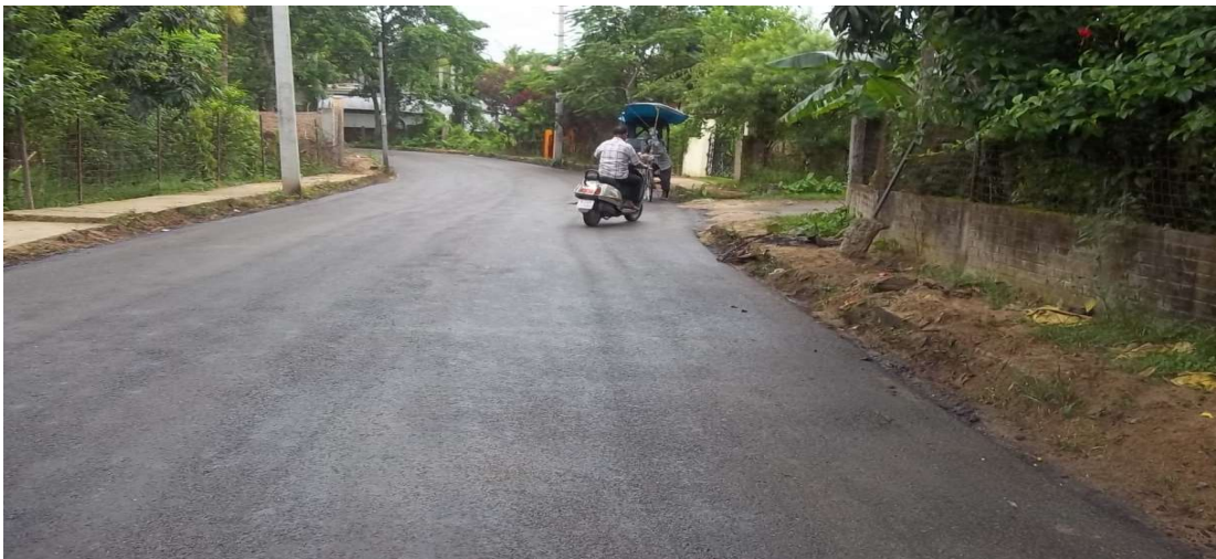
Fig 13: Completed Cold Mix SDBC Road.
