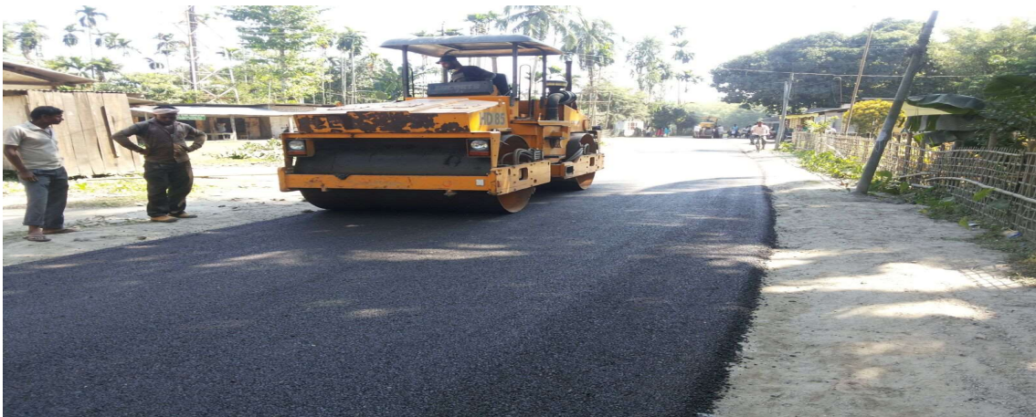
Fig. 10: Compaction of cold mix CGPC by roller
