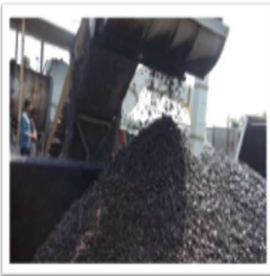
Produced Cold Mix®s getting collected at the Tipper
