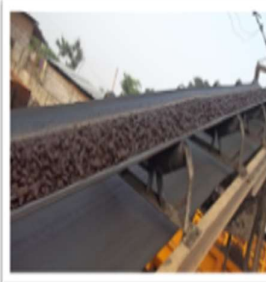
Produced Cold Mix® is being carried through conveyor belt
